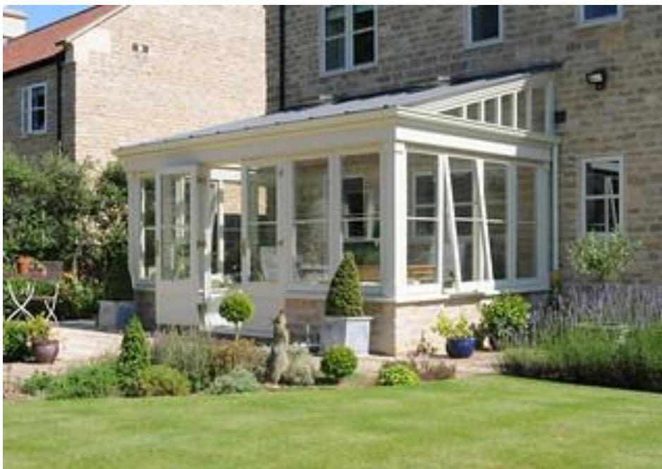
Figure 14: Rear extension- Image courtesy of www.davidsalisbury.com via flickr
